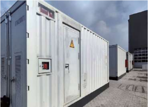
BRES Vehicle Certification Lab Project Country: Germany
