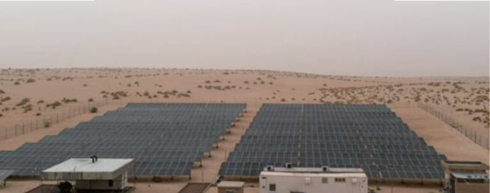
Niger light wood storage project Country: Niger Configuration: Lithium battery system: 1224kWh PCS: 600kW PV: 600kW
