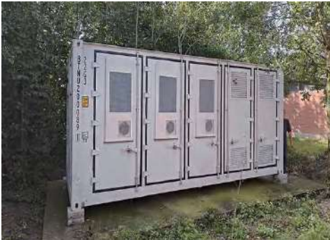
20ft BRES Pig Farm Project Country: Belgium
